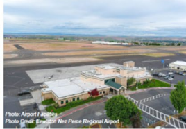
Photo: Airport Facilities Photo Credit: Lewiston-Nez Perce Regional Airport
