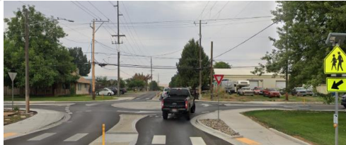
Figure 2 – RRFB at 10th Street and Burrell Avenue.
