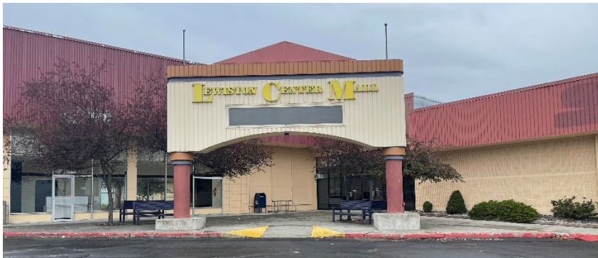
Figure 2.32. Lewiston Center Mall as viewed in April 2023 was identified as a potential area of change.
