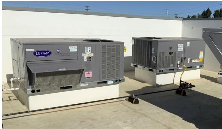
Proposed HVAC System – Typical Packaged Roof-Top Units
