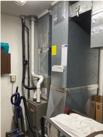
Existing Gas-Fired Furnace and Overhead Air Distribution
