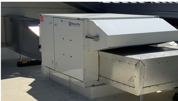
Proposed Ventilation System – DOAS Unit (left) with Heat Recovery Core (right)
