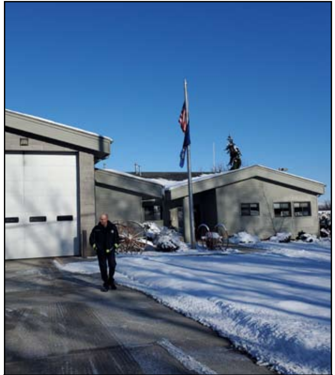
STATION 2: SOUTH SIDE ENTRANCE Public Entrance.
