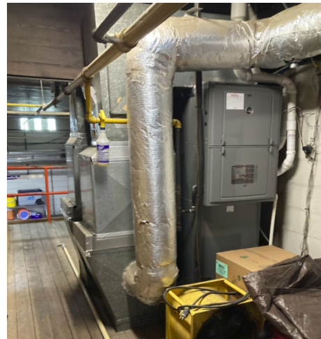
Existing Gas-Fired Furnaces, Filter Banks and Outside Air Intake Ducts (wrapped)
