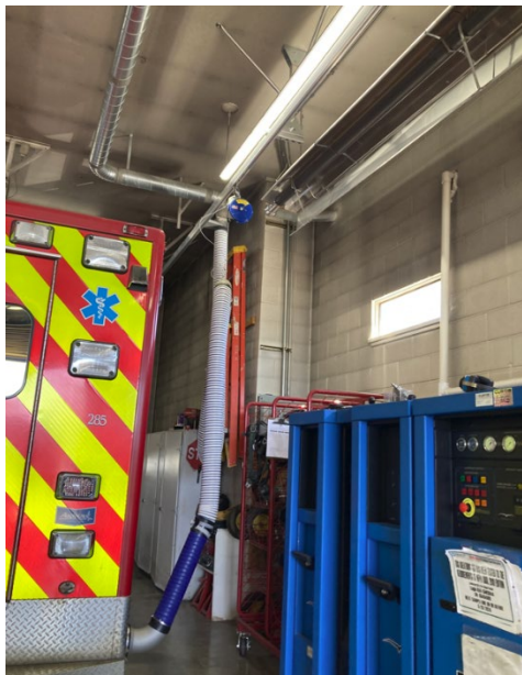
Existing Apparatus Bay Tailpipe Exhaust and Radiant Tube Heaters
