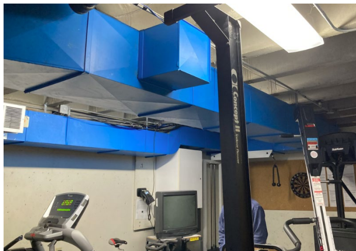
Existing Basement Fitness Area and Exposed Ductwork
