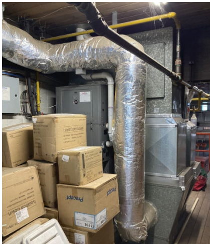
Existing Gas-Fired Furnaces, Filter Banks and Outside Air Intake Ducts (wrapped)
