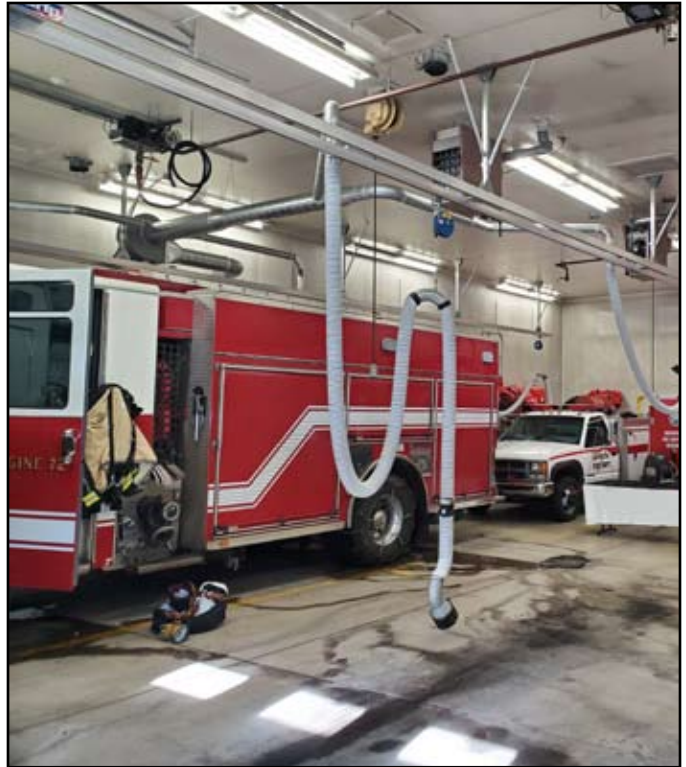
STATION 2: APPARATUS BAY Poor floor drainage. Vehicle exhaust provided. No general exhaust.
