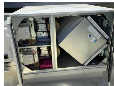
Proposed Ventilation System – DOAS Unit (left) with Heat Recovery Core (right)
