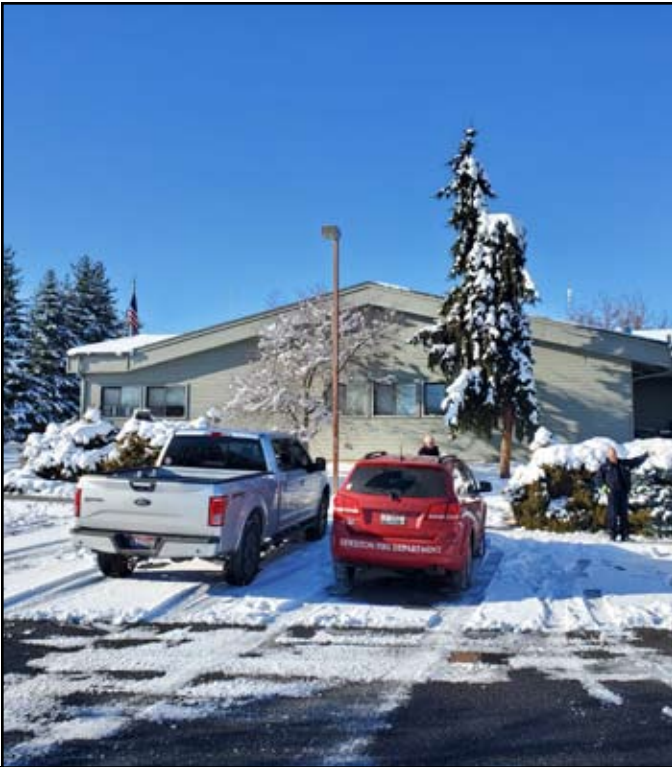
STATION 2: EAST SIDE PARKING Limited staff parking.
