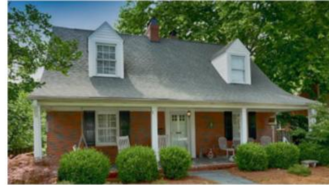
full facade porch
