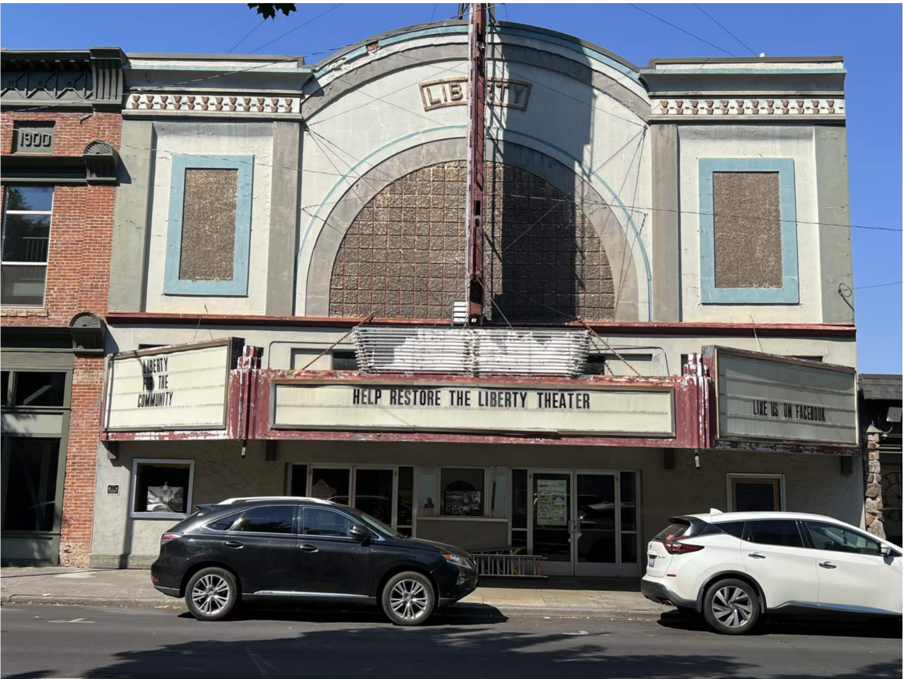
FRONT FACADE - EXISTING CONDITION EXISTING 4-LINE READER BOARDS AND UNORIGINAL CENTER LIBERTY SIGN
