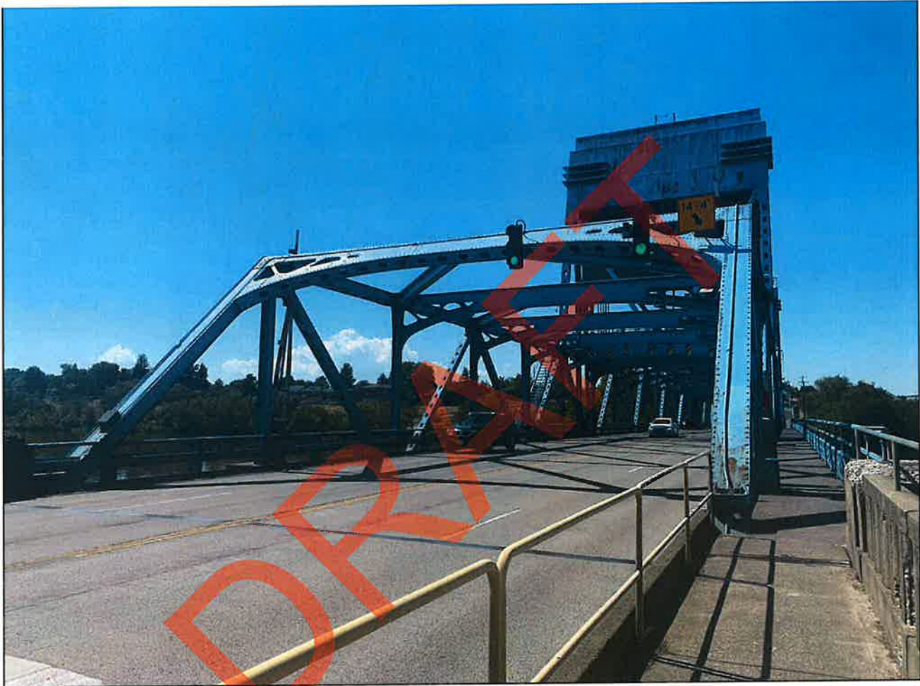
Photo 8. View looking west from the northeast end of the bridge.
