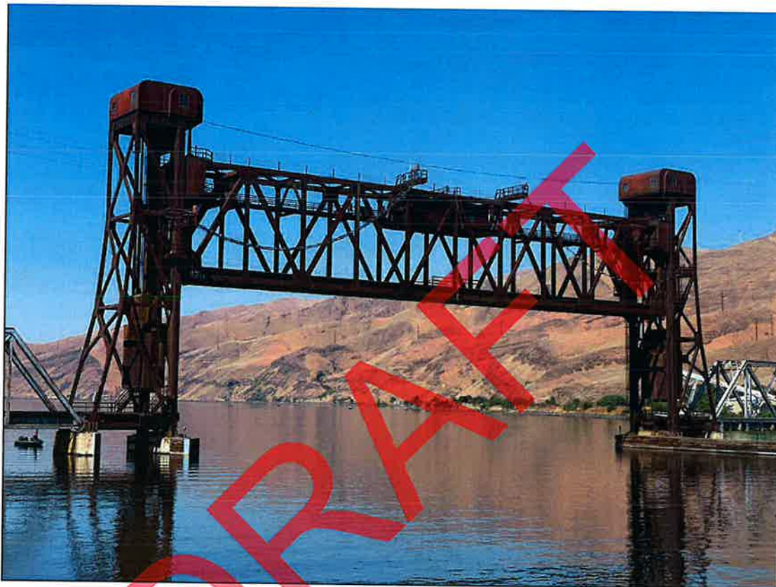
Photo 2. View looking northwest at the vertical lift span of the bridge.
