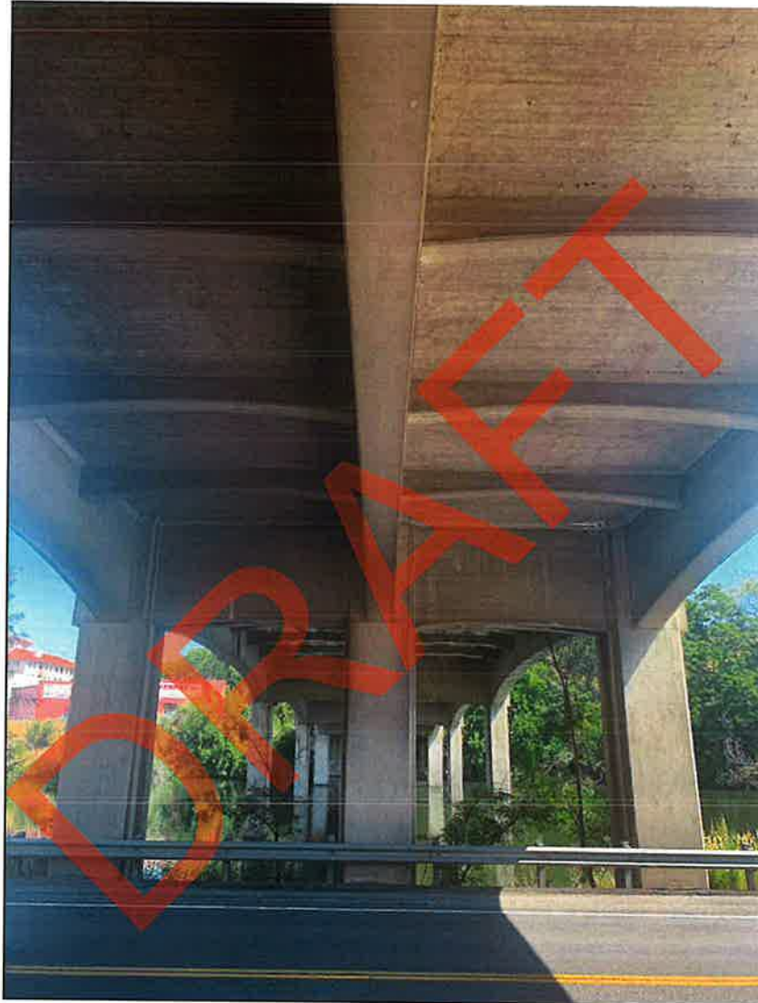
Photo 5. View looking east under the east end of the bridge.
