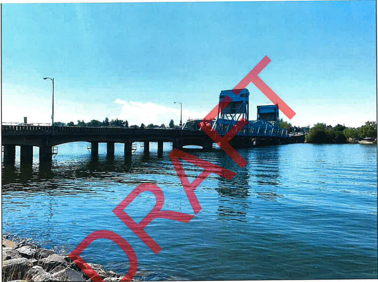
Photo 6. View looking west from the east end of the bridge.
