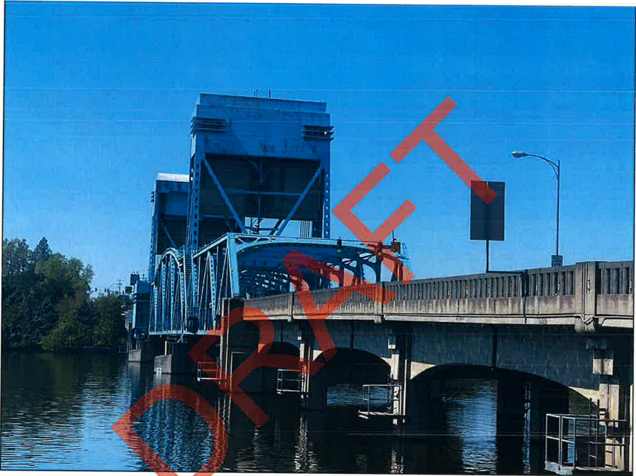
Photo 3. View looking west at the bridge.
