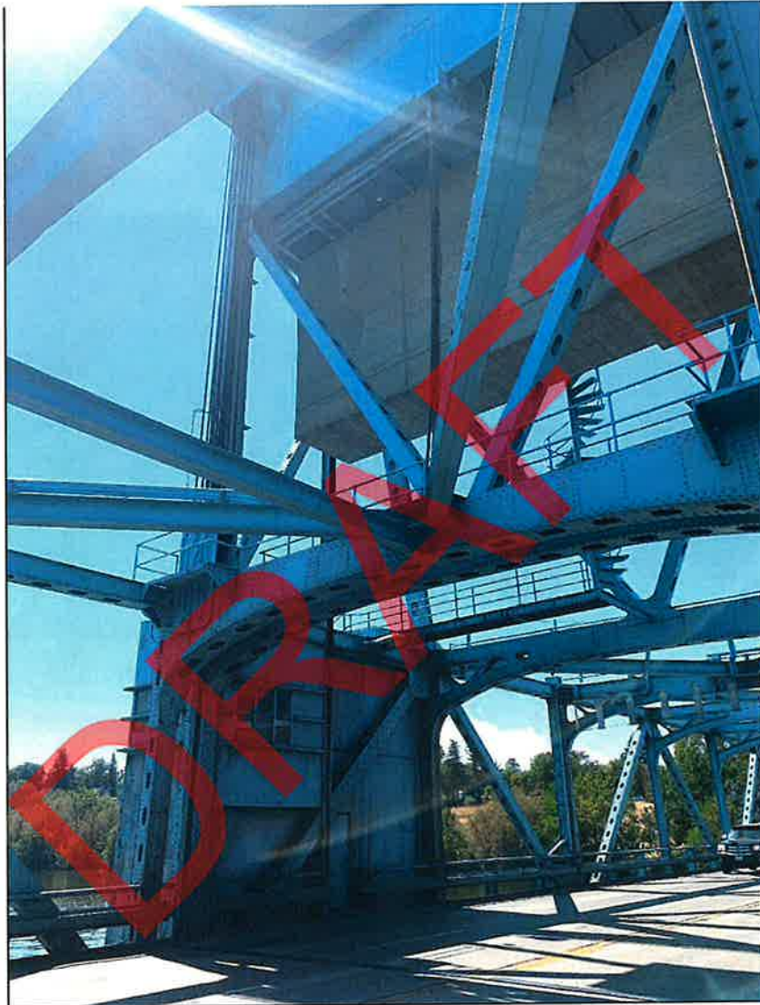
Photo 10. View looking at the operator's house on the south side of the western tower and the counterweight of the vertical lift span.
