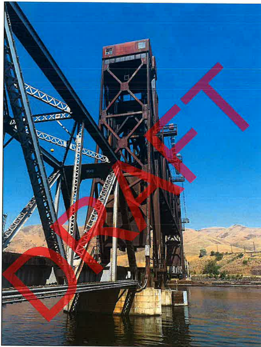
Photo 4. View looking north at the piers, Warren truss span and vertical lift span.
