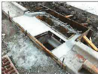
"Drop Inlet" during construction
