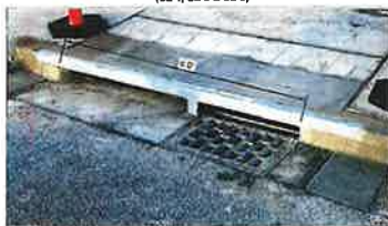
Completed "Drop Inlet"
