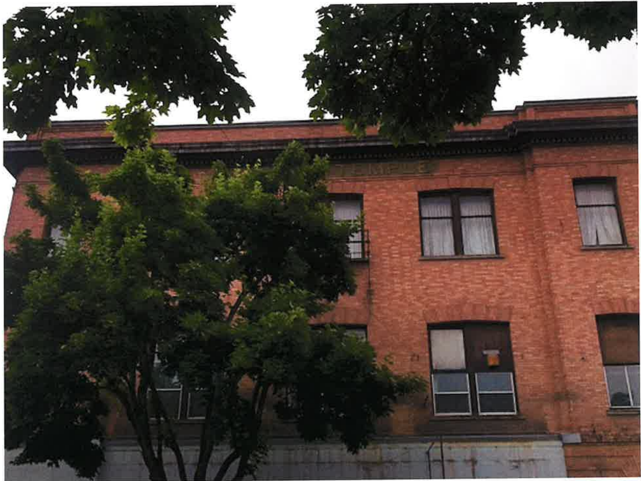
Windows to be replaced or painted
