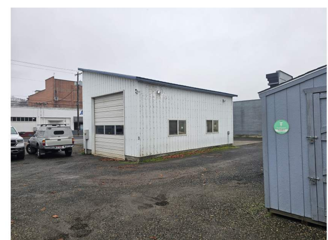
EXISTG PHOTOGRAPH PROVIDED BY OWNER - NORTHEAST PERSPECTIVE
