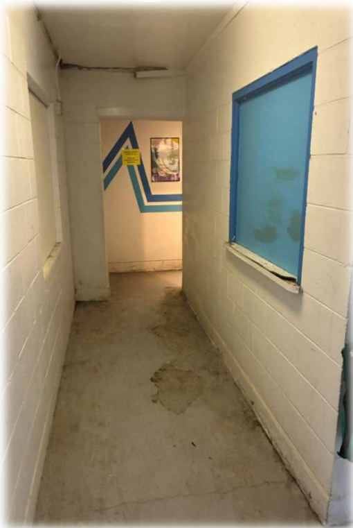
Hallway facing men's changing area
