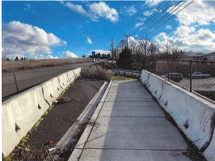
Figure 5 Looking South next to Regence BlueShield just before 23rd Avenue.
