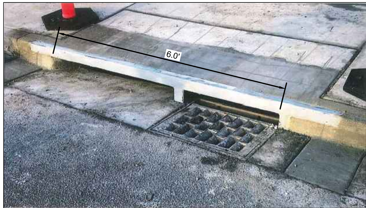
Completed "Drop Inlet"
