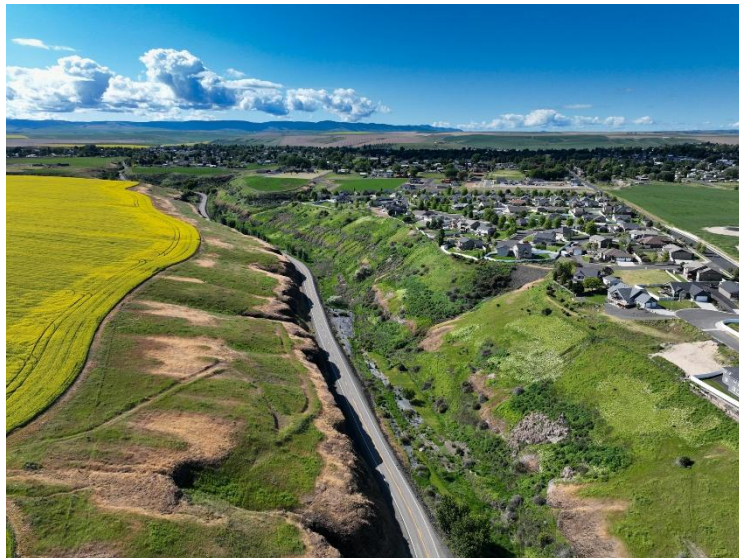
Connecting to Lindsay Creek Road is particularly challenging due to the steep topography and creek.
