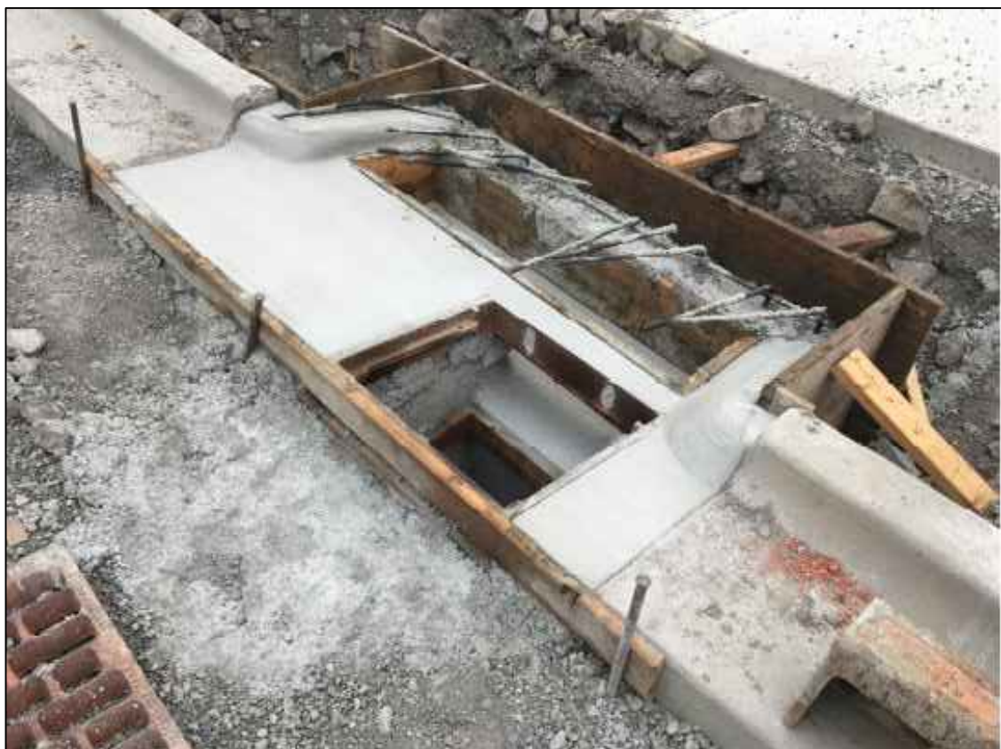
"Drop Inlet" during construction
