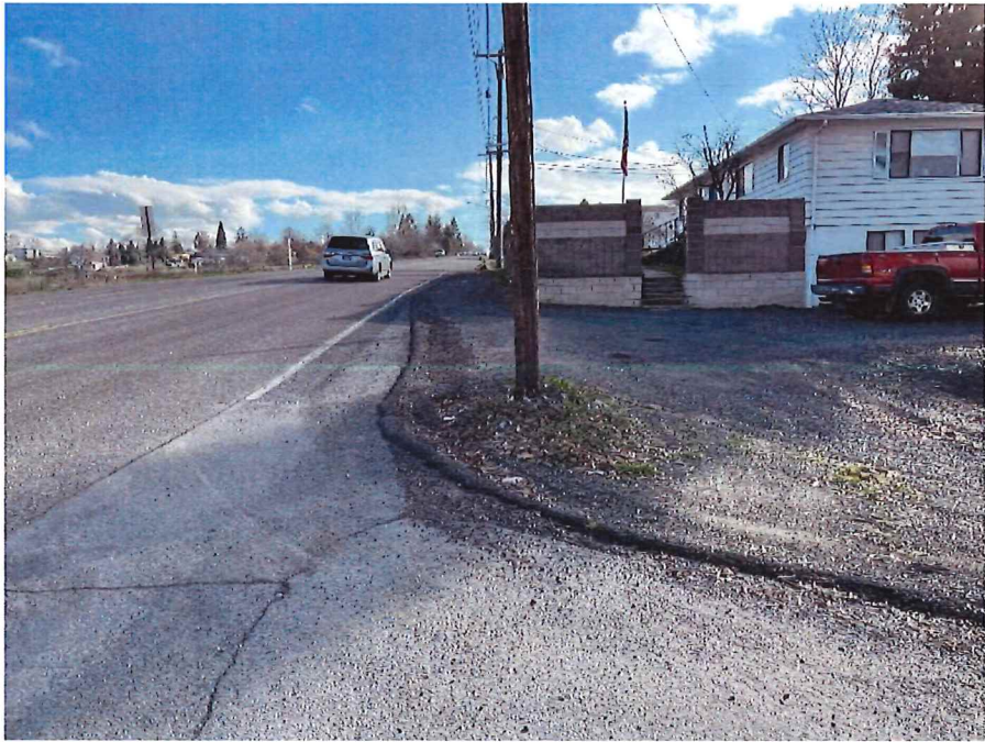
Figure 6 Looking South from Vineyard Drive.
