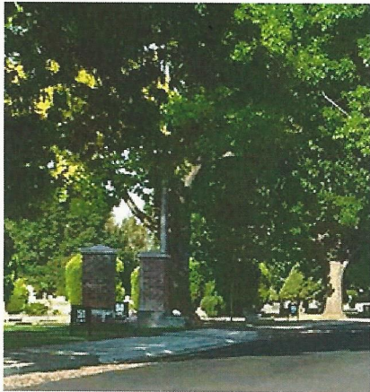
Figure 33: Existing Pillars at Entries, Source: LEES+Associates.
