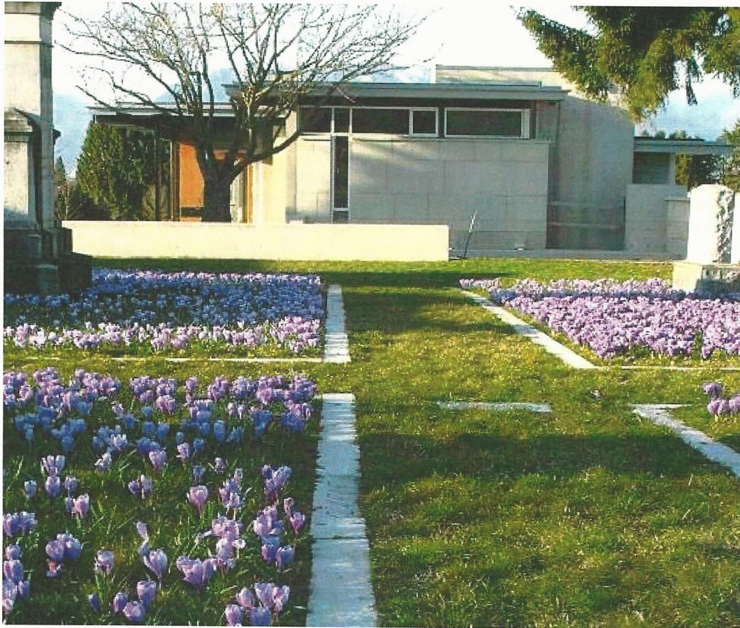
Figure 15: Mountain View Cemetery Customer Service Building and Celebration Hall, Vancouver, British Columbia. Source: LEES+Associates.
