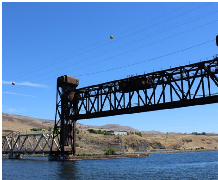
Figure 5: Railroad lift span bridge over the Clearwater River.
